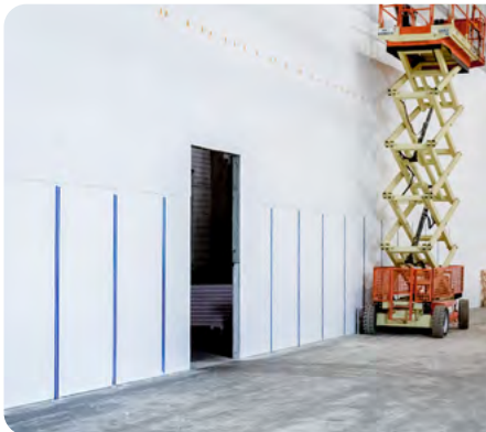
RamPanel prepared with blue tape for HygiSeal 3.1 installation.
