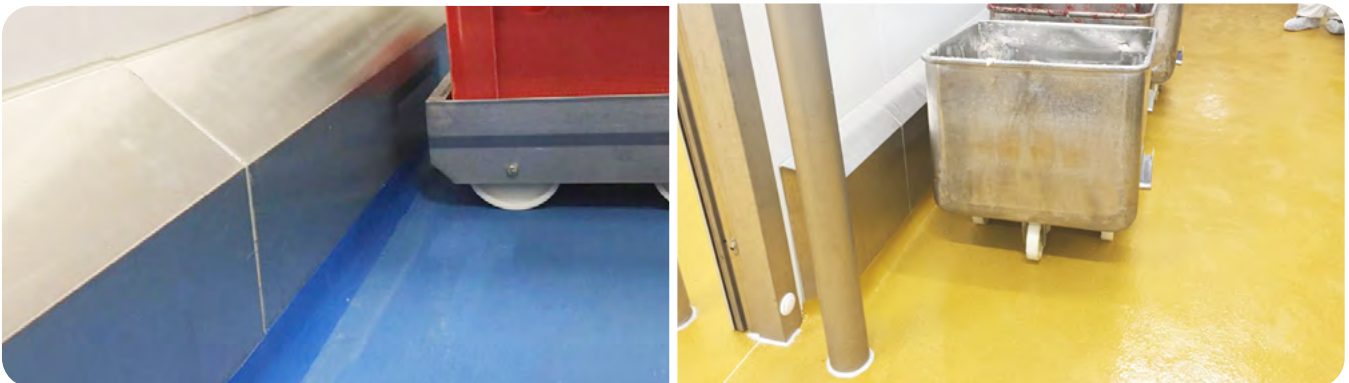
PolySto prefabricated ICS40RB stainless steel kerb with concrete core with a resin floor applied into the rebate.
