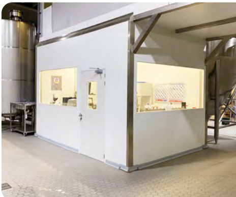
Brewery laboratory build with HygiWall .
