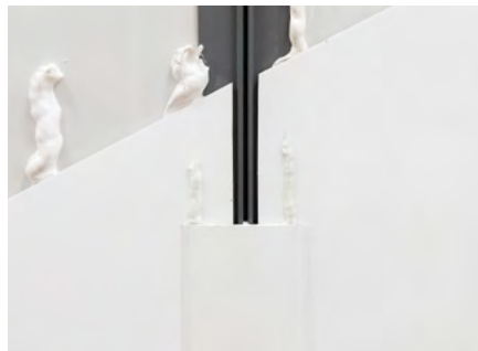
CleanSheet finished with PVC profiles.
