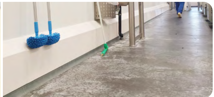
PolySto prefabricated IP40RB SaniCoat CleanRock kerb with a resin floor applied into the rebate.
