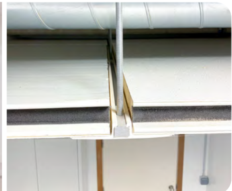
HygiWall ceiling suspension (Aluminium T-profile).
