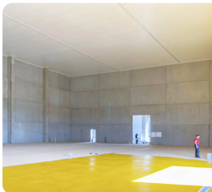
RenoPanel as hygienic ceiling in a potato processing facility.
