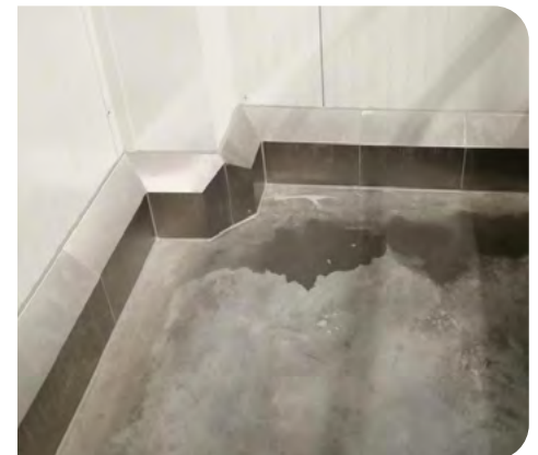
PolySto prefabricated ICS30R stainless steel kerb with concrete core.
