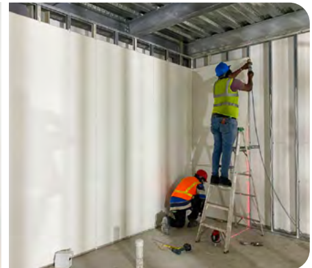
RamPanel can be installed on metal studs.
