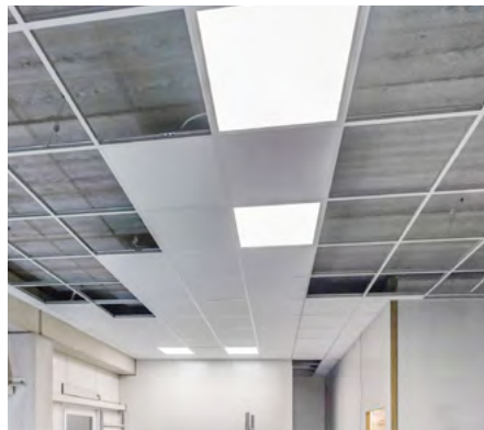
Installation of HygiCeiling.
